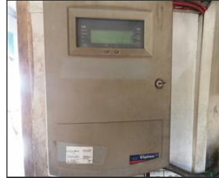
Photo of non-conformity Finding 7.14 Fire alarm system found inactive.JPG
