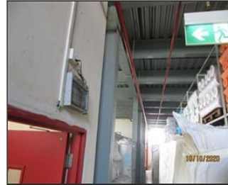
Photo of non-conformity Finding 7.14 No illuminated exit sign has been posted on the fire door.JPG
