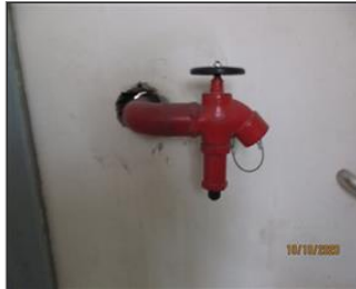
Photo of fire safety equipment Fire Hydrant point at production floor.JPG
